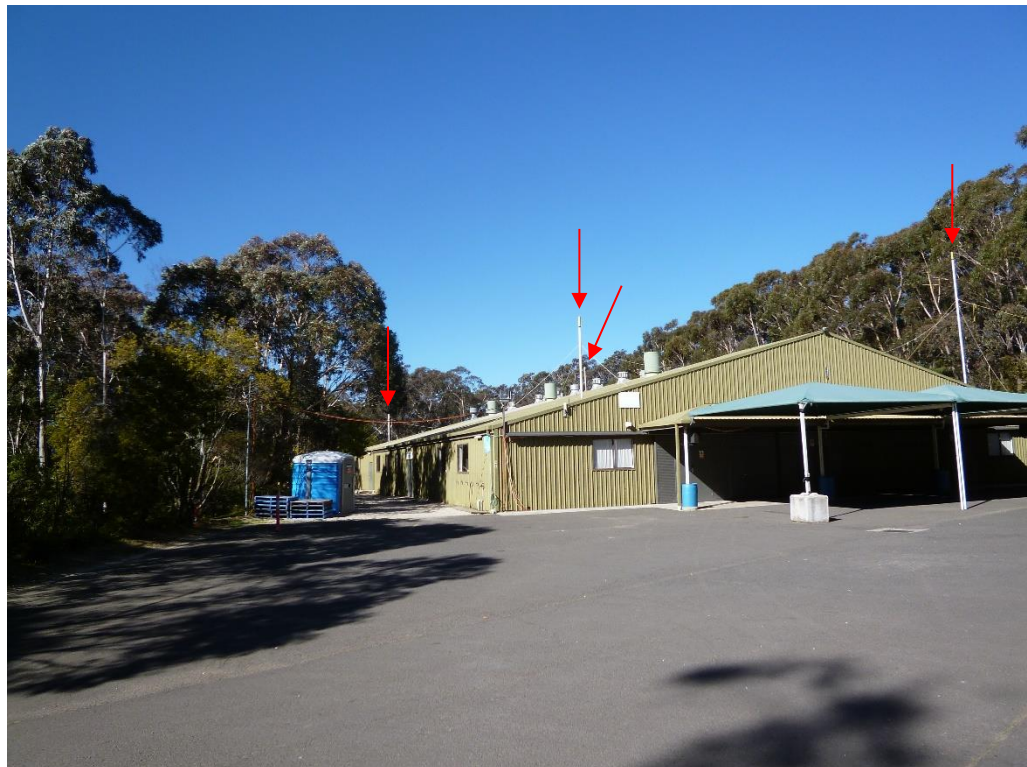
Figure 1 Height Poles installed at location of proposed auditorium. Height poles indicated by red arrows
