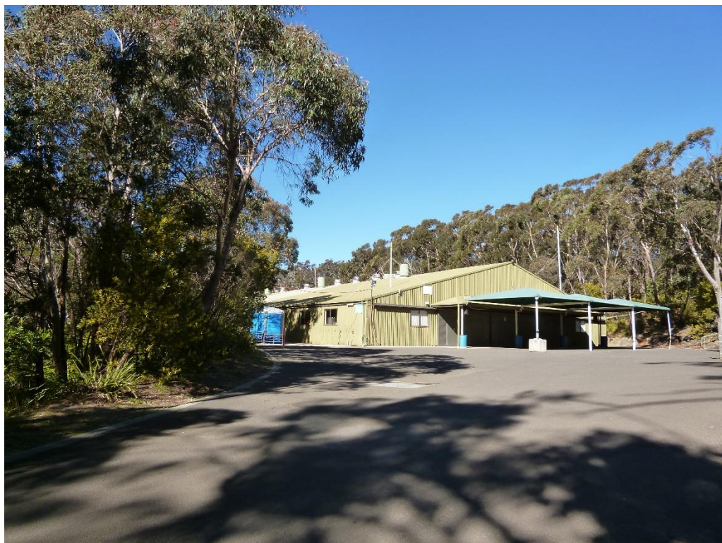
Figure 6 Existing KCC auditorium building with height poles installed
